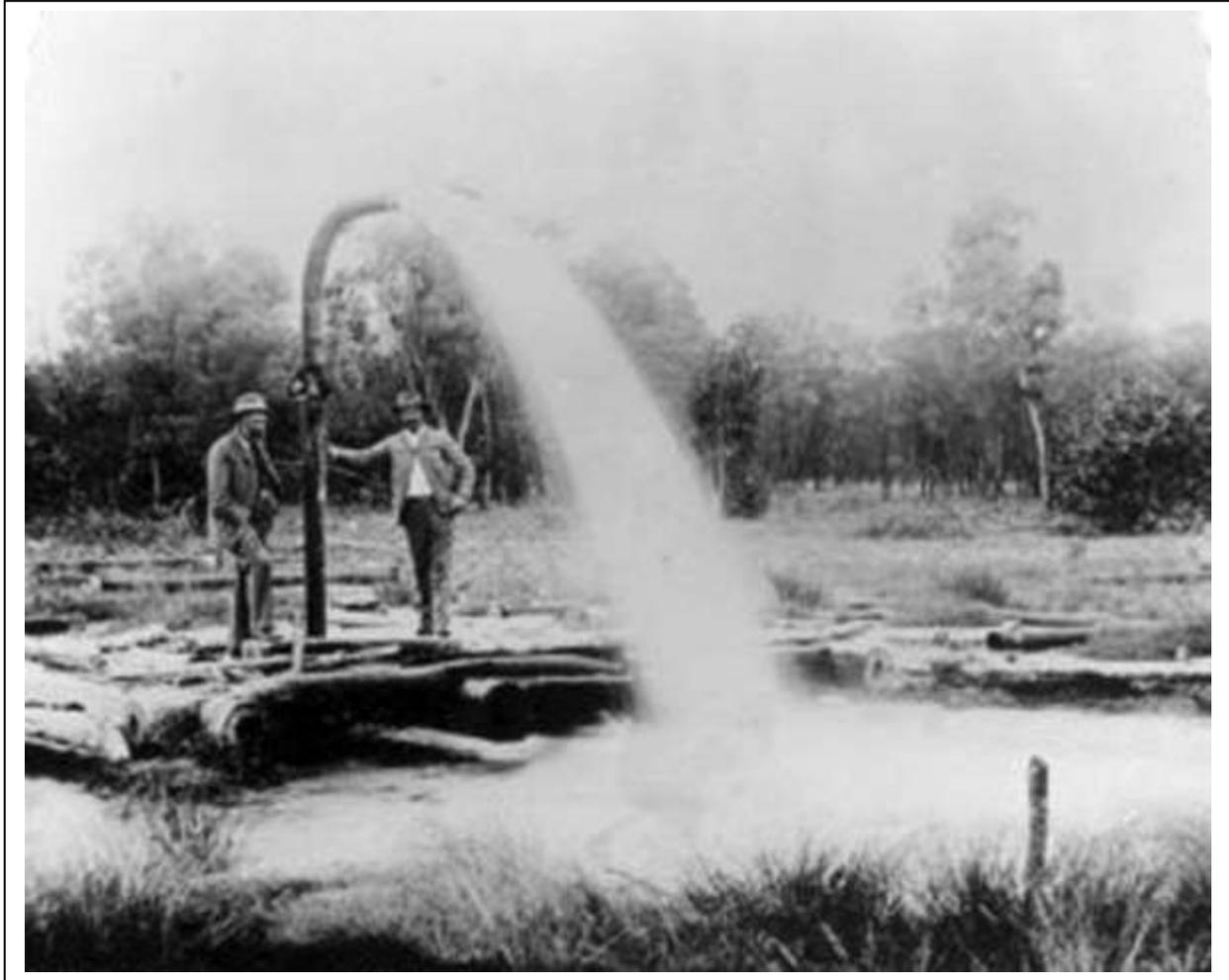
*Bore at Murweh station 1890, depth 548 metres and gave 83,000.000 Litres per 24 hours*
