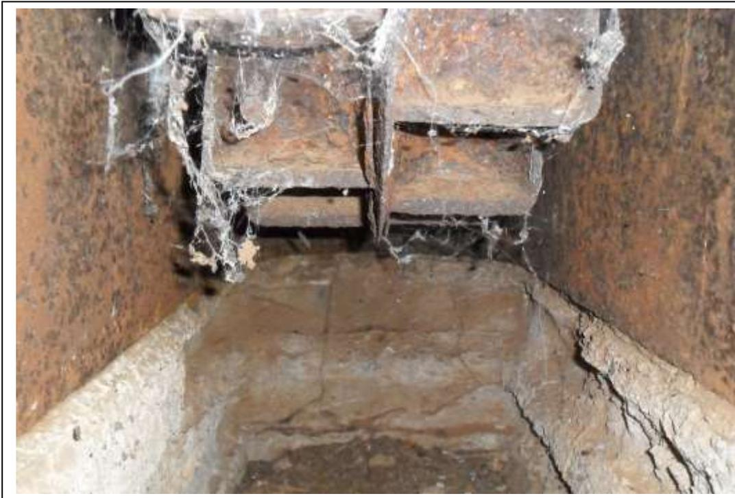
*Photo of the vanes within the Pelton wheel unit at Warrambah Station
