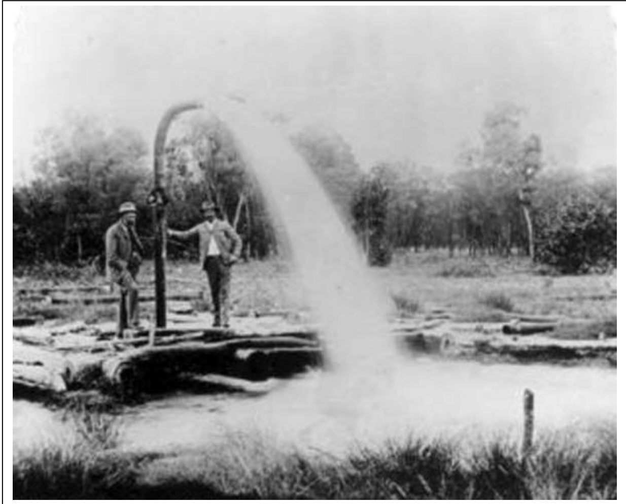
Bore at Murweh station 1890, depth 548 metres and gave 83,000.000 Litres per 24 hours
